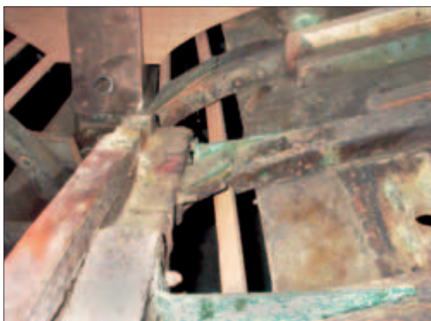
Corroded engine beds
