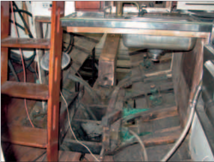
Under the galley obvious corrosion spot
