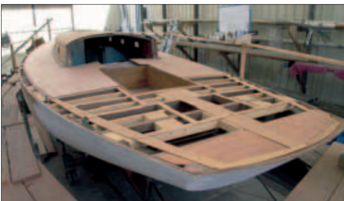
New decking and beams
