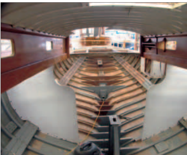
New frames and floors
